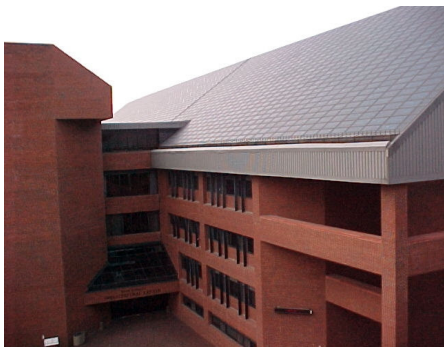
30,000 SF Solar Roof in Washington, DC
